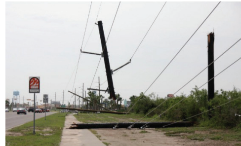
Figure 2-11. Downed Power Lines
