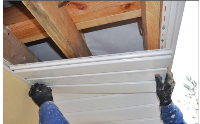
Figure 3-15. Soffit Bracing
