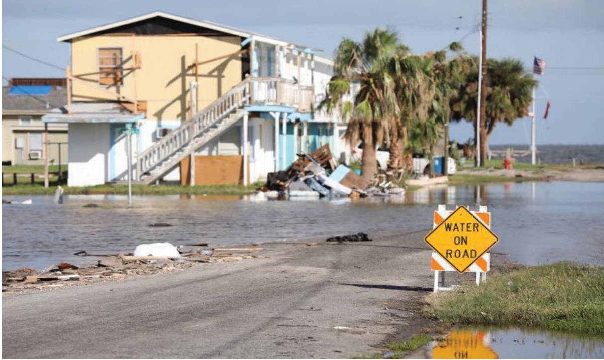
Figure 1-14. High Tide Flooding in Rockport, TX. Photo by Chip Van Zandt
