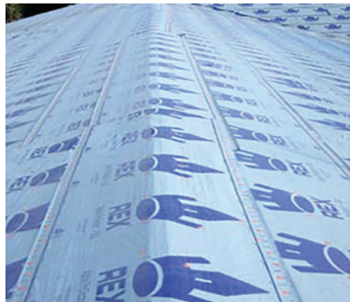
Figure 3-9. Synthetic Roof Underlayment Source: IBHS
