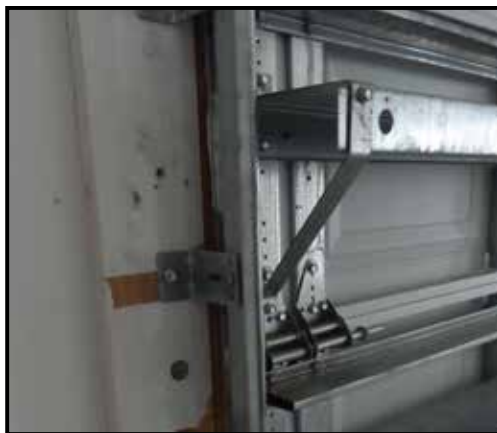
Figure 4-20. Fortified Garage Door. This replacement garage door is fortified with heavy duty metal bracing on every panel and stronger brackets connecting it to the door frame.
