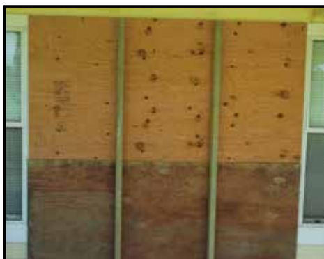
Figure 4-19. For larger windows, such as this sliding glass door, two 2x4s face outside and are oriented with the narrow end against the plywood. The fastening screws attach from the plywood into the 2x4.
