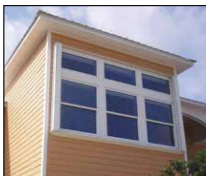
Figure 4-9. Accordion shutter (shown in open position) installed over a large window group of a coastal home. Shutter has been installed to allow deployment from inside the home.
