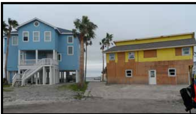
Figure 4-22. Two Neighboring Homes in Aransas County after Hurricane Harvey. The elevated house on the left received no damage, while the at-grade house on the right has been boarded up due to extensive damage.
