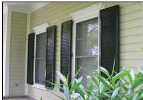
Figure 4-11. Colonial shutters made from durable extruded aluminum components add a traditional look to the home and protect window openings.
