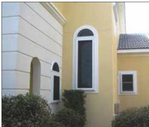
Figure 4-14. In-place stainless steel impact screen protecting several windows of a coastal residence. This system requires no deployment and provides shade.
