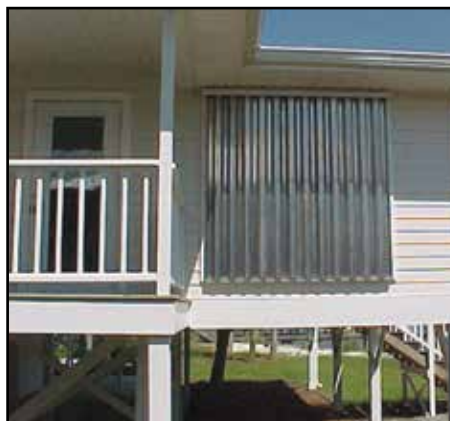
Figure 4-13. These 0.050 gauge aluminum storm panels offer cost-effective storm protection. In this example, panels slip into a track above the window and secure onto a bottom track using wing nuts.
