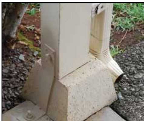
Example of Retrofitting. Here, a metal strap connects the vertical post to the foundation, which finishes the continuous load path from the roof to the foundation.
