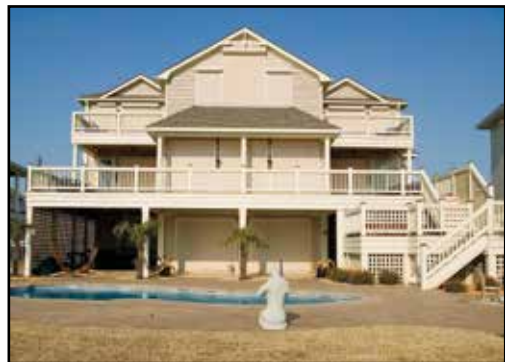
Figure 4-8. Coastal home protected with roll-down shutters on all windows and doors. The shutter is held in place by vertical guide tracks and can be deployed manually or with an integrated electric motor.
