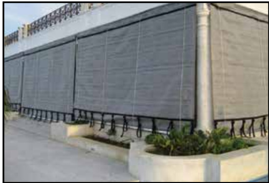
Figure 4-16. Polyethylene basket-weave fabric windscreen is deployed at the edge of a patio, enclosing the entire area.
