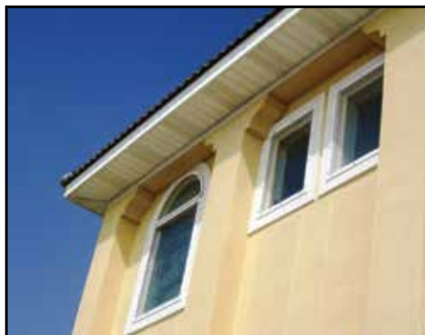
Figure 4-15. Flat impact polycarbonate panels are installed directly over windows of a coastal home. This window covering provides excellent storm protection with minimal aesthetic impact.
